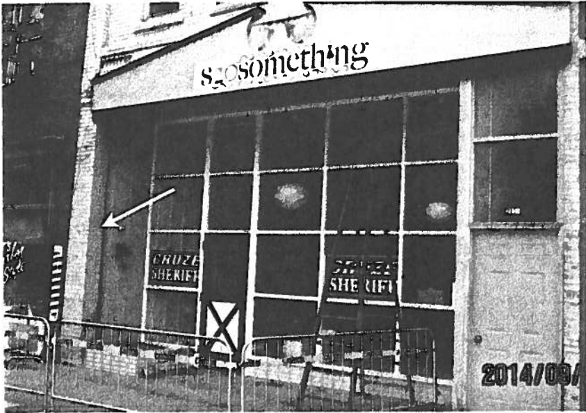
First floor of Palm Building West column shown with arrow
