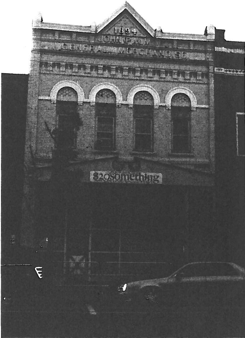
John Palm Building c. 1894 215 Sibley Avenue North Litchfield, MN
