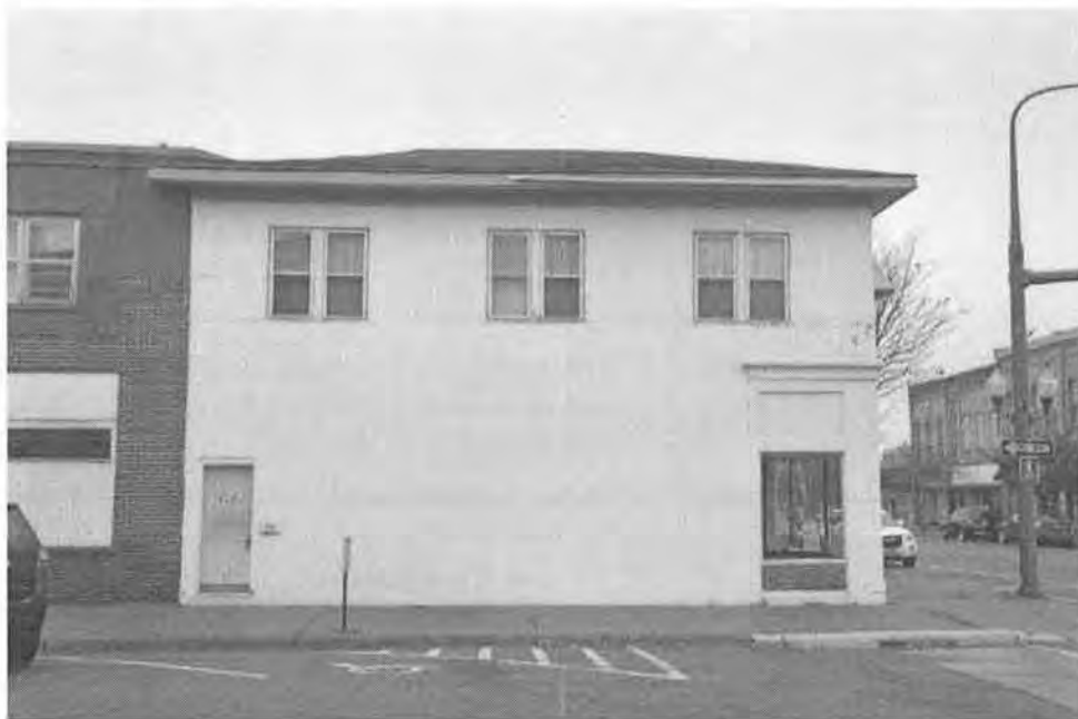
Photo 4. The north facade (2017, facing southeast).
