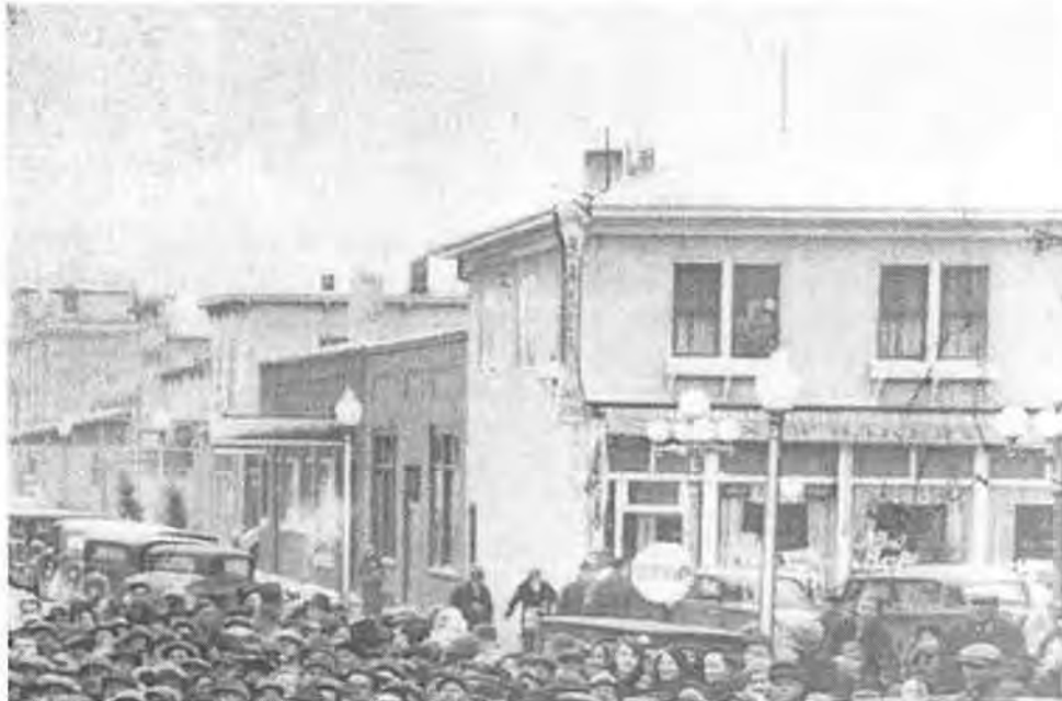
Photo 1. Circa 1934 view of the building (detail from a photo owned by the Meeker County Historical Society, Litchfield).
