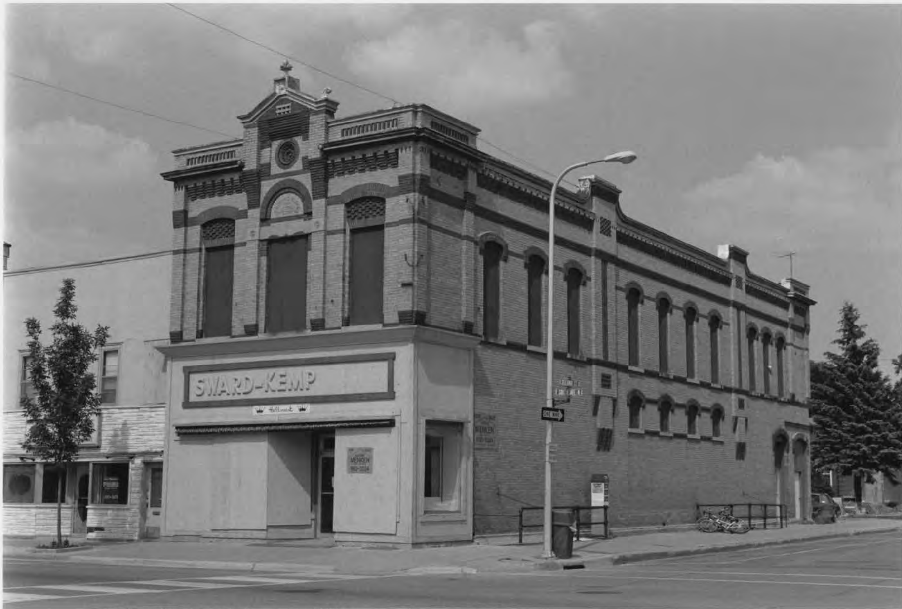
Brown Block, 202 N. Sibley Ave. Litchfield Commercial Historic District Meeker Co., MN Old 578-22
