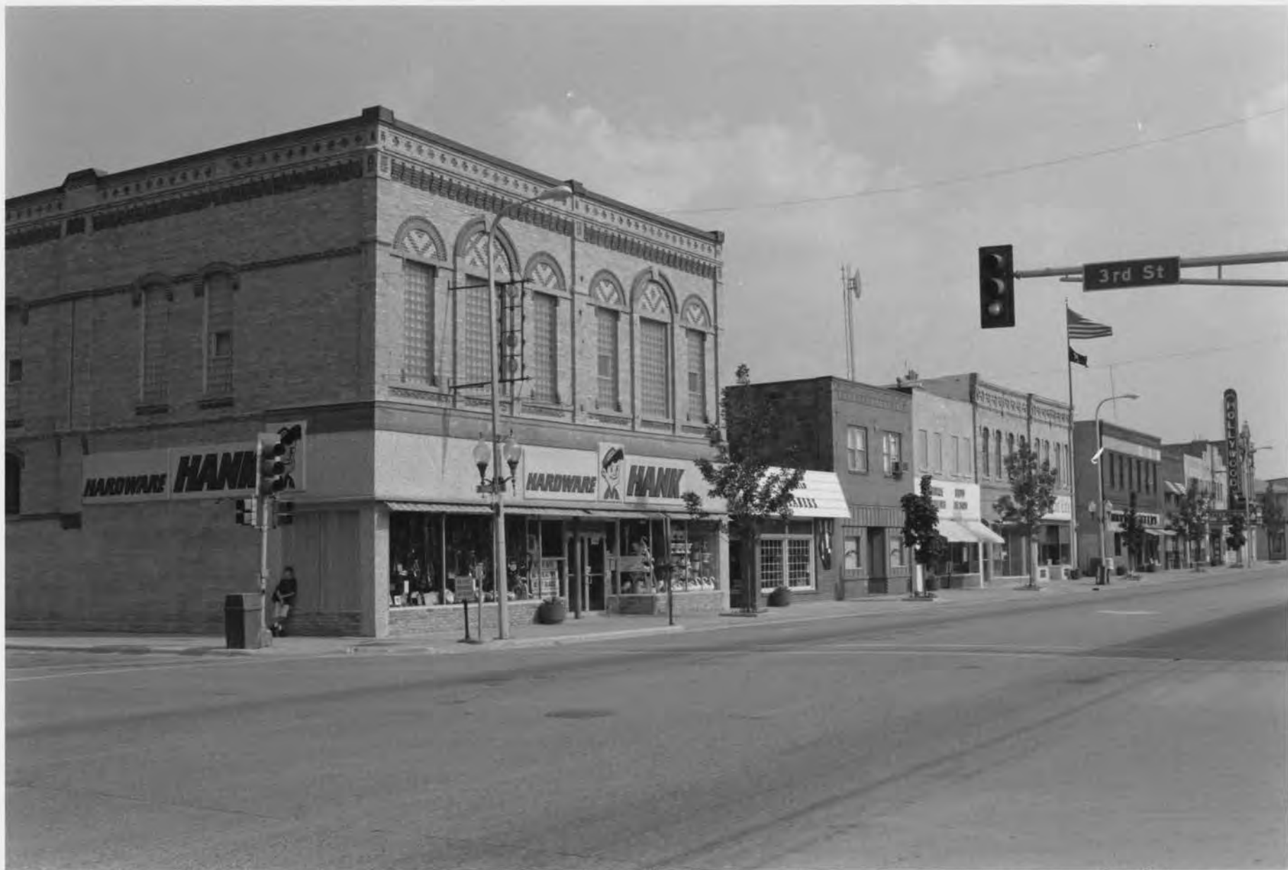
Streetscape: Looking SE at East side of Sibley Ave. #242 is on left. Litchfield Commercial Historic District meeker Co., MN 012576-4A
